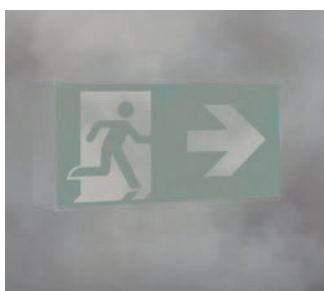
Badly illuminated escape sign
