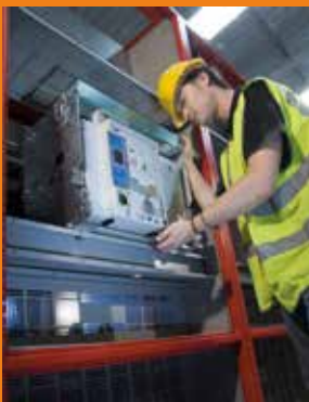
Direct Response Engineer Installing Retrofit ACB
