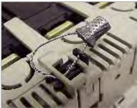
Terminal Cover Lock with Lead Seal
