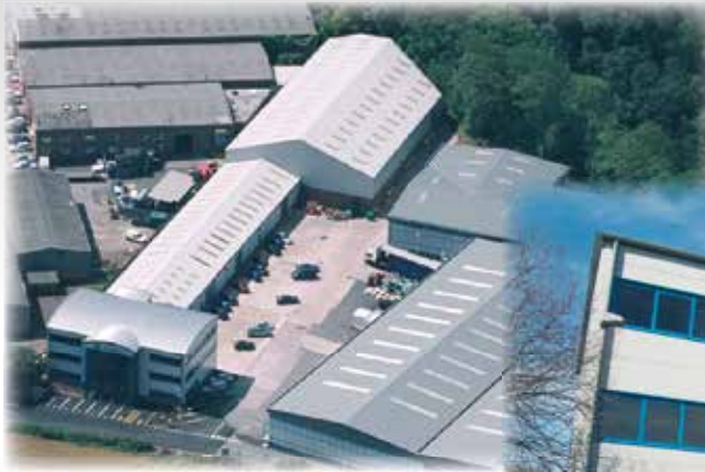
Cembre Ltd. factory in Curdworth (Birmingham)
