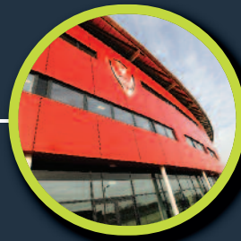
Installed in a host of prestigious sites
