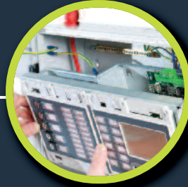
20 way earth bar and lots of working space
