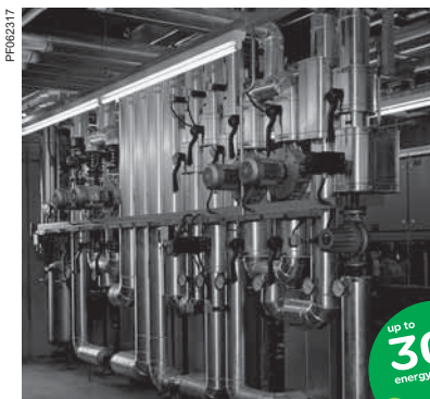
ATV 12 controlling a pumping station
