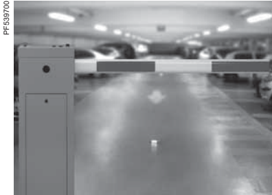
ATV 12 controlling an access barrier
