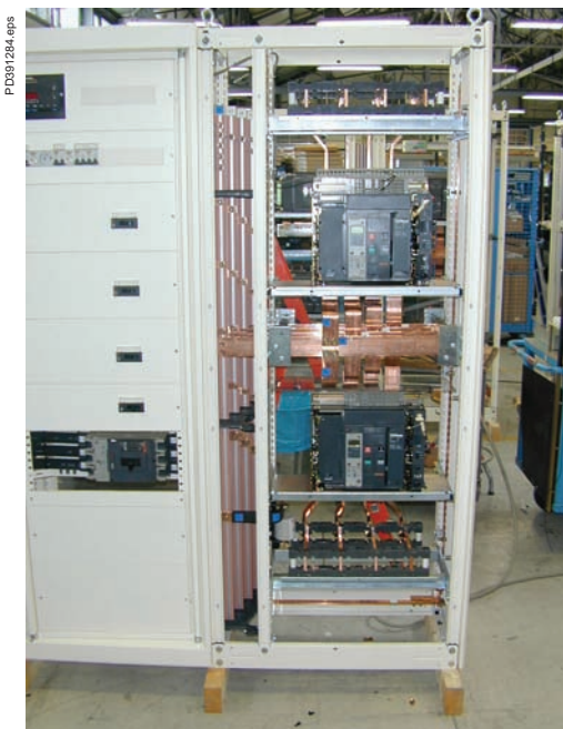
Source changeover system in 2 combined cubicles.
