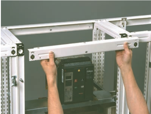
Cross-pieces can be removed to facilitate work.
