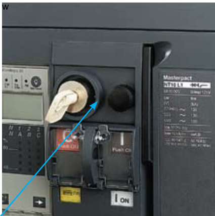
Electrical closing pushbutton BPFE.
