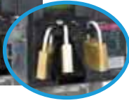
Rotary handle locked by a keylock.
