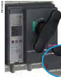
Rotary handle locked by a keylock.
