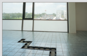
Completed Soluflex installation
