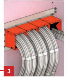
3 Modular plates allow for increased capacity
