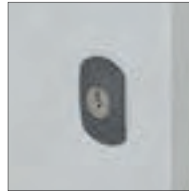
Internal doors accept key barrel
