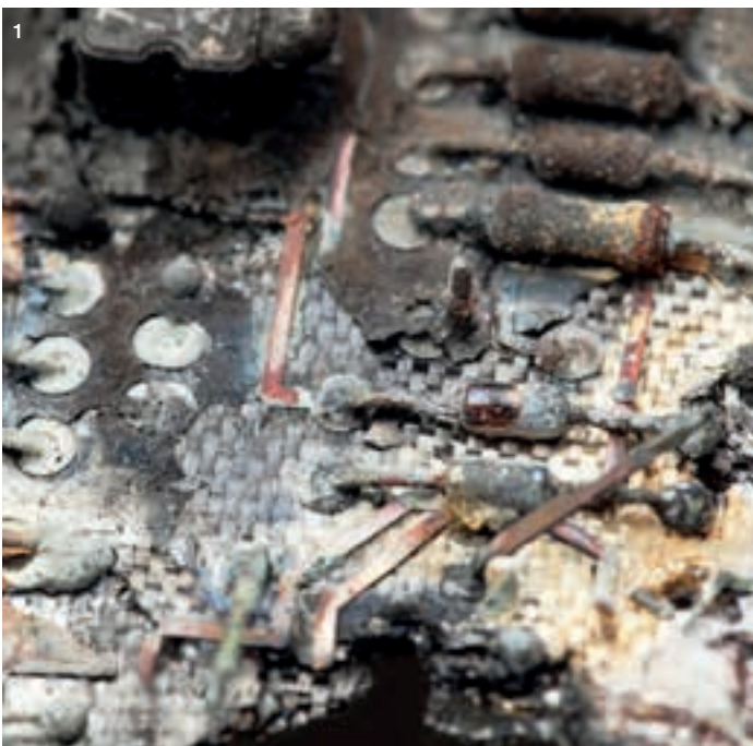
1 Transient overvoltage damage to a circuit board | 2 Most damage is barely visible
