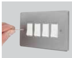
Finally after decorating, fit the cover plate.
