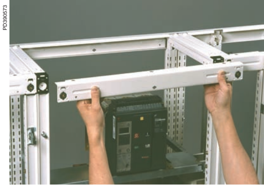
Cross-pieces can be removed to facilitate work.
