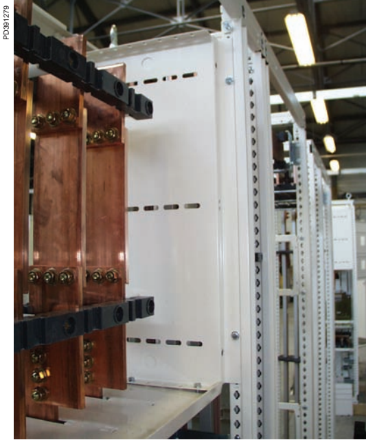
Dismountable vertical busbars.
