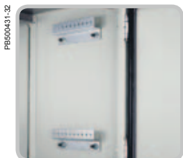
Perforated rails installed on lateral studs.
