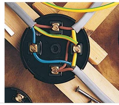
The requirement for accessibility applies equally to the situation where, because of damage to an existing cable, a repair is effected by the introduction of a joint.
